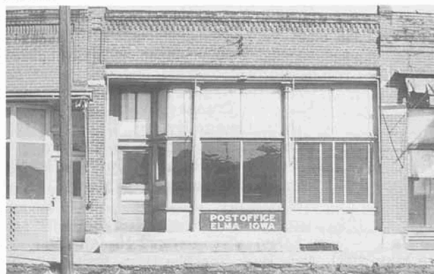
Elma Post Office on east side of town.
