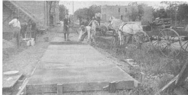
Ebert Brothers laying sidewalk in front of the Brick Flats.
